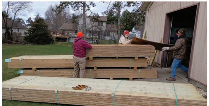
A team of Rock County Chapter volunteers move stacks of lumber donated by JP Cullen for use on future structures. Photo by Dennis James.
